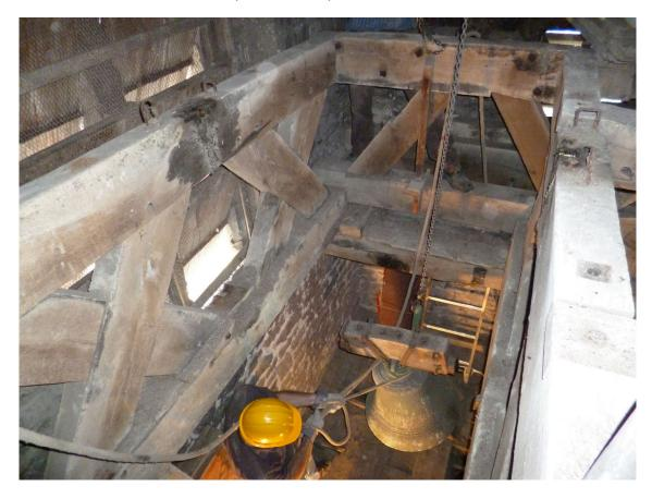
The unringable ring of eight bells has been replaced with a True Harmonic cast ring of bells in a new metal bellframe. The back three bells of the new ring were originally part of the chime at the now demolished church of St Mary (RC), Highfield St, Liverpool. Bells from the old ring have been relocated at Sydney (Dulwich Hill), Ipstones, Willingale and Prescot.
