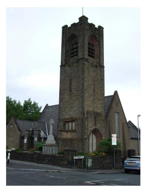
An ambitious project to restore the eight-bell chime and hang the bells for traditional full circle ringing has been completed. The chime framework had badly rusted causing damage to the tower and bell installation. The four smallest bells have been replaced by larger bells cast to ringing weights.
